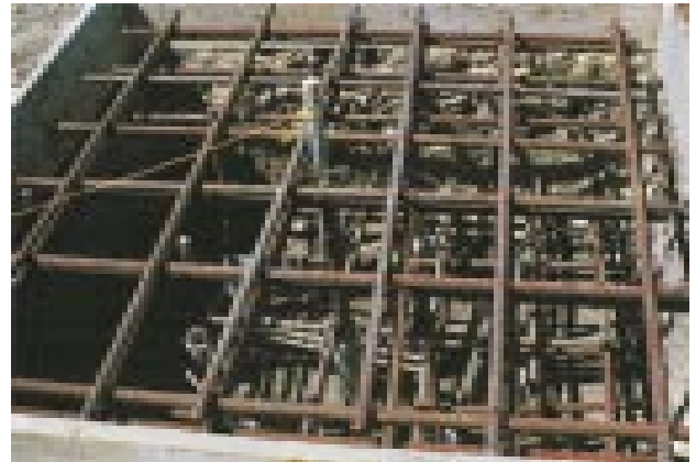
• Twelve HS piles and rebar for tower mast
