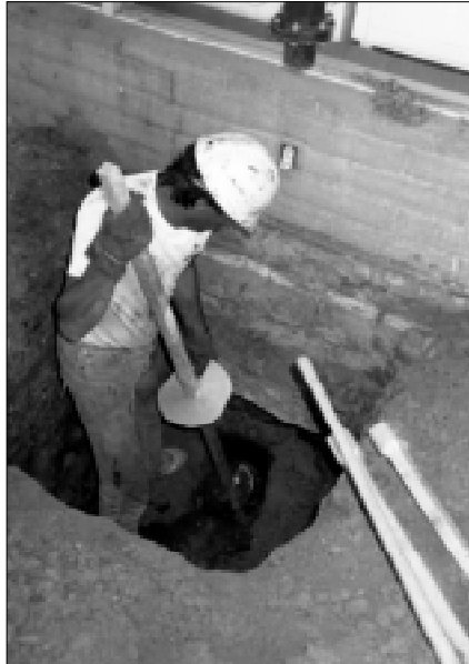
Anchor being spotted next to foundation
