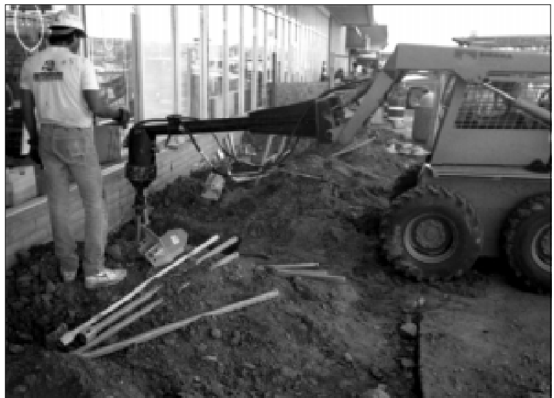
Skid loader driving screw anchor to 40'
