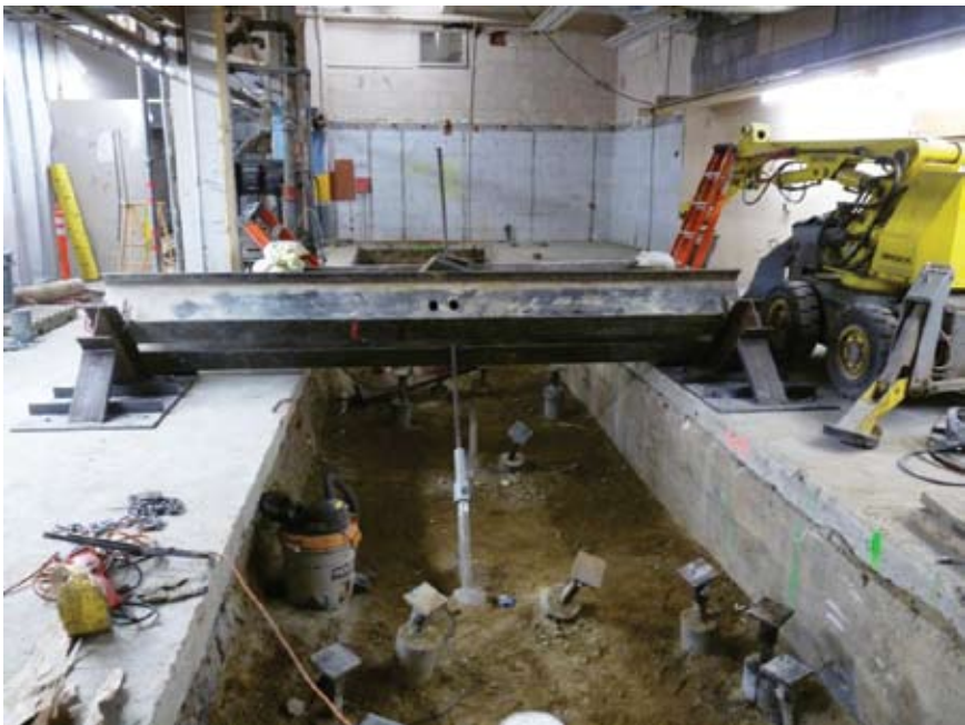
Proof testing the 45-degree battered piles to 117 Kips.
