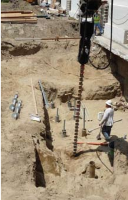
Above picture compares the relative ease of augering outdoors with the drill head on an excavator versus the special equipment and effort this job required for its indoor confines.
