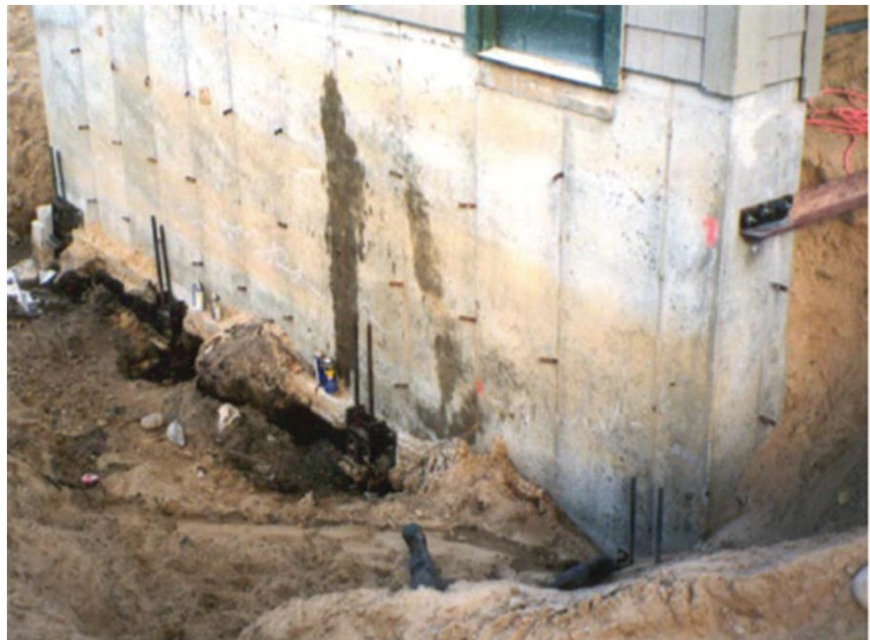
Above, side of the garage showing installed piers No. 1, 2, 3 and 4.
