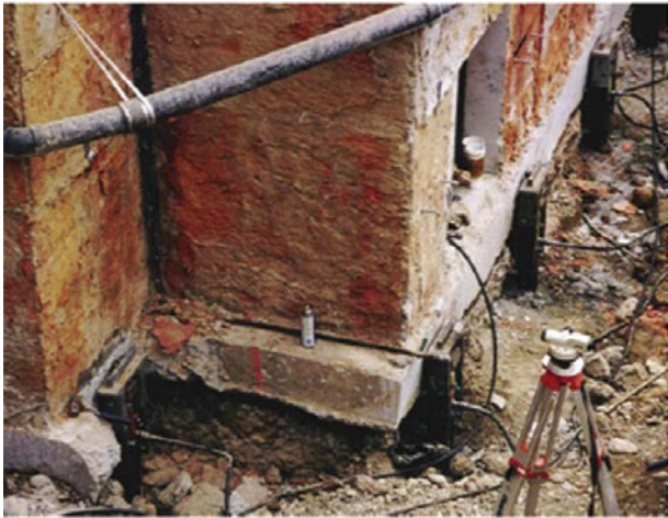
The photographs above show Atlas Resistance® Piers with hydraulic rams attached during the restoration of the structure. Notice the photo at right shows a lift of over 2 inches at the window well.
