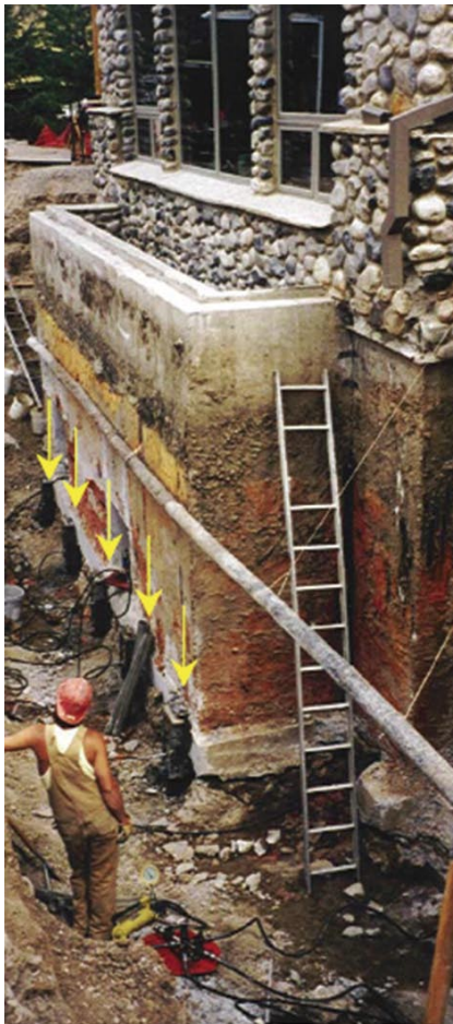
Photograph at left shows the excavation to expose the footing. Notice the installer mounted five Atlas Resistance® Piers to the stem wall for the window wells near the great room.
