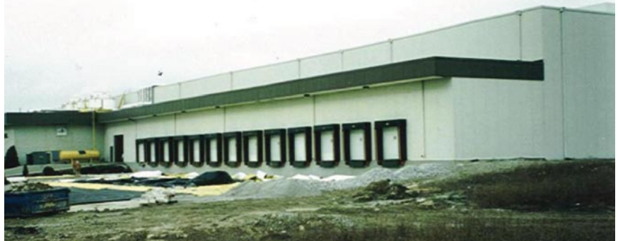
This is a view of the front of the structure. The loading dock shown here had settled 8 inches. Some areas at the right side of this building suffered settlement in excess of 22 inches!
