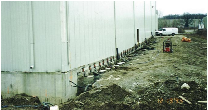
The photo above shows the right side being carefully and gently lifted. Note the hydraulic rams on each pier.
