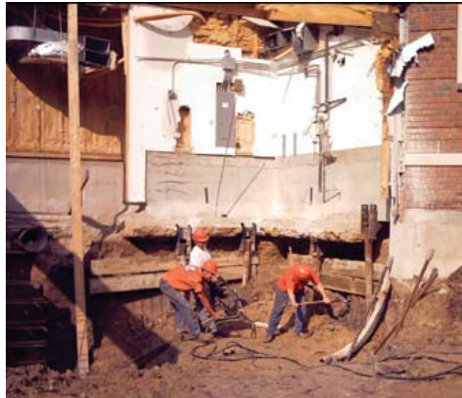
Adding an extension to a helical tieback anchor
