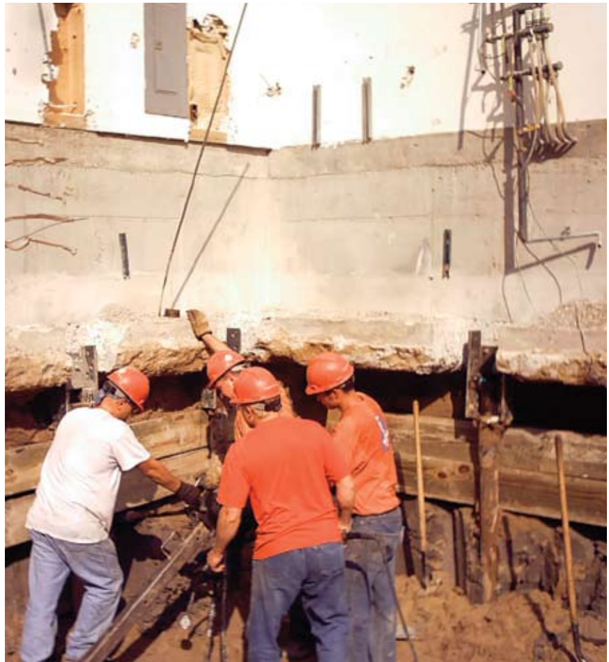
Installing CHANCE® helical tieback anchors between Atlas Resistance® piers
