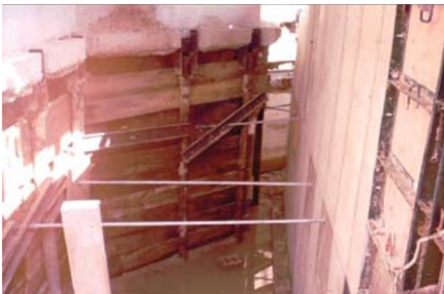
Tieback anchor rods extended to steel walers for lateral support during basement wall construction
