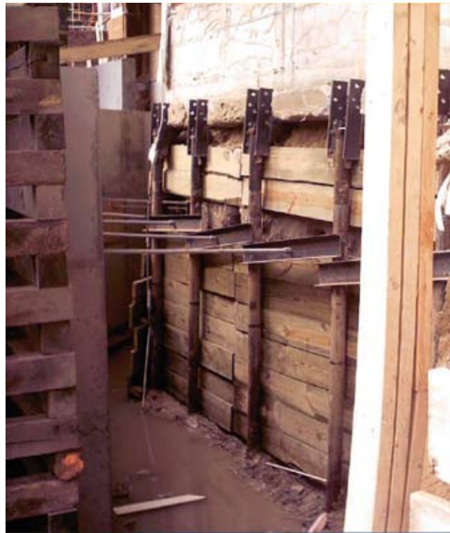
Tieback anchor rods extended to steel walers for lateral support during basement wall construction
